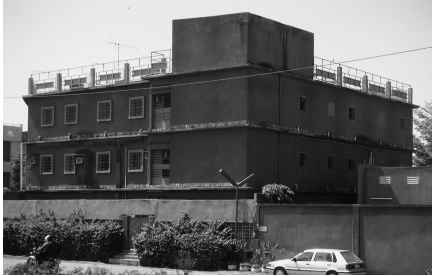
FIG. 5. Downtown structure used for building-scale heat storage measurements.
