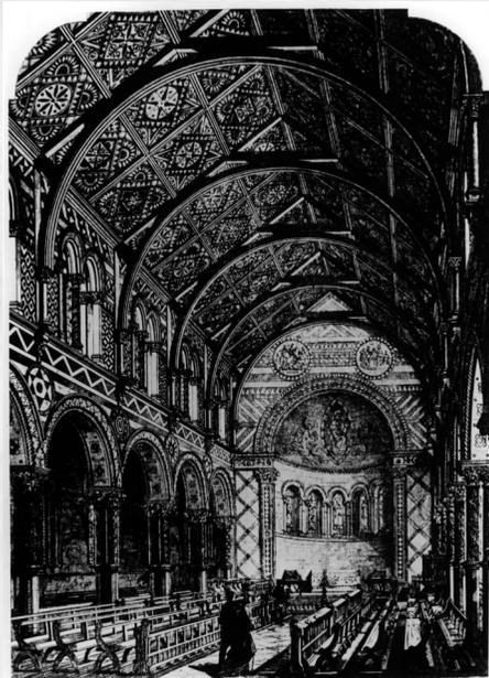
As the Chapel is situated above the Great Hall, Scott had to overcome a number of structural difficulties. He had to use a light-weight construction system for the arcade and upper nave walls that concentrate the loading above the iron columns on the floor below. The wall is therefore fabricated in iron with paired ornamental cast iron columns and an applied timber frame facing above. The original roof was lightly built in order to reduce stress on the wall framing.
