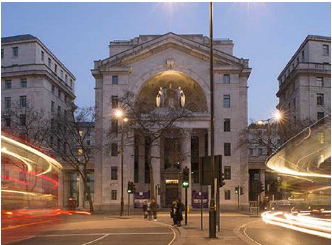
1. Bush House looking south down Kingsway
